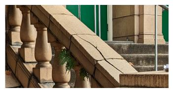
TC-3 - Significant cracking at main entry balustrade cap
