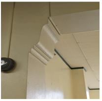
Figure 3.37.3- Plaster molding detail at locker bay
