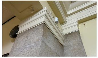
Figure 3.34.5 - Ornamental plaster pilaster cap
