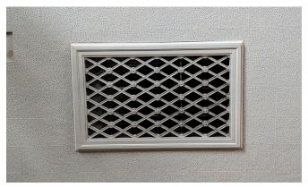
Figure 3.36.1 - Plaster ceiling grill with surrounding acoustical treatment
