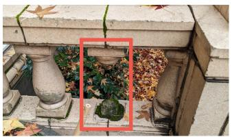
TC-6 - Heavily damaged baluster at front entry.
