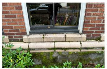
*BC-1* - Cleaning at brick, terra cotta, and concrete to remove atmospheric soiling and bio-growth.
