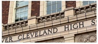
Figure 3.7.2- Mortar joints at main entry cornice displaying typical staining.
