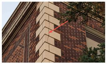
Figure 3.7.3 - Cracked terra cotta units at southwest building corner.
