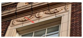
TC-6 - Non-historic steel lintel installed above window at front entry.
