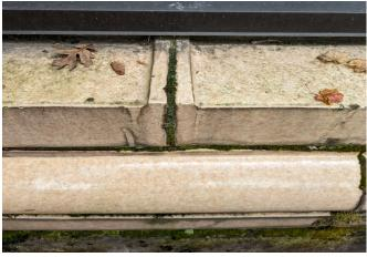
TC-1 - Soiling at terra cotta window sill joint
