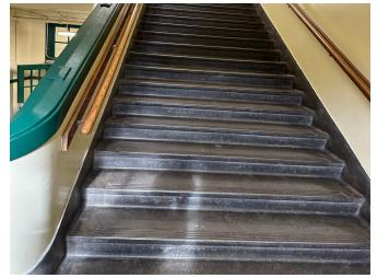
Figure 3.38.2 - Typical cement stair risers with inset metal safety treads.
