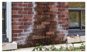
*B-2* - Deteriorated mortar joints at roof overflow outlet.
