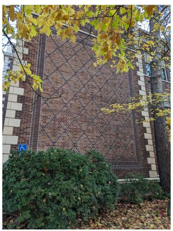
Figure 3.4.2 - Diamond brick pattern at north end of West Elevation
