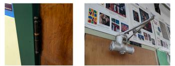
Figure 3.27.1- Original hinges (left) typically remain. Closures have been replaced, with the exception of one potbelly closure (right) found in the old gym.
