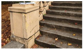
TC-4 - Glaze spalls and chips visible at base of main entry balustrade
