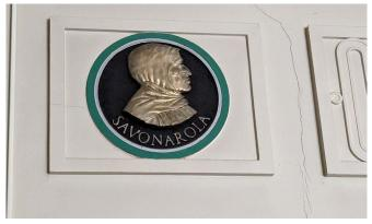
Figure 3.36.3- Ornamental plaster figure head, showing adjacent cracking.
