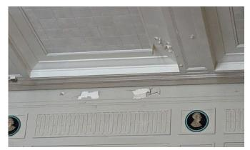
Figure 3.36.2- Water damage at ceiling and wall.
