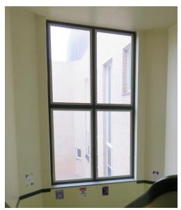
Figure 3.20.1- Vinyl sash replacement window at courtyard stairwell
