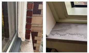
*Figure 3.19.1 - Original exterior brickmold at aluminum replacement window (left); original marble stool at interior (right).*
