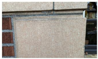
*Figure 3.7.1 - Typical observed condition of terra cotta at quoin units, showing crazing at glaze.*
