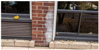
E-2 - Chalk residue visible at North elevation.
