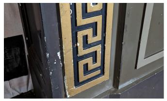
*Figure 3.35.3 - Minor damage at proscenium arch ornamental plaster.*
