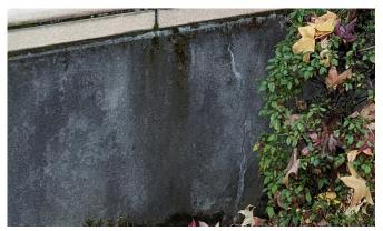
C-2 - Bio-growth and cracking at parge coat
