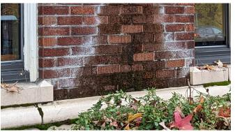
*E-1 - Efflorescence below roof drain overflow outlet.*
