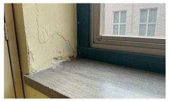
*Figure 3.19.3 - Vinyl sash replacement window, displaying potential water infiltration damage.*
