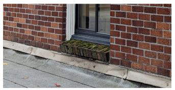
E-4 - Heavy bio-growth soiling at brick window sill joints
