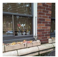
Figure 3.25.1- Obsolete wiring through brickmold
