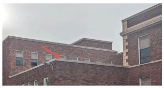
Figure 3.15.2 - Sheet metal cap flashing visible at parapets
