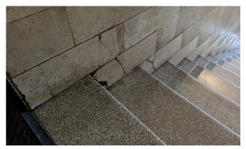
Figure 3.34.1- Cracking at marble wall base
