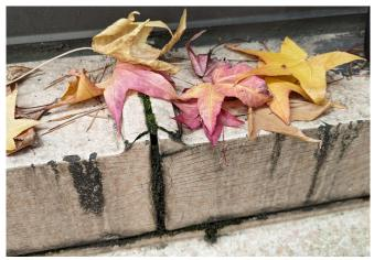
TC-2 - Minor cracking at T.C. window sill joint.
