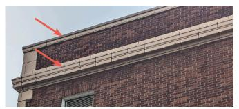
Figure 3.6.2 - Terra cotta cornice and parapet cap with metal cap flashing.
