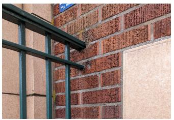
*B-1* - Original railing connection at Brick. Brick replacement will be required if railings are removed.
