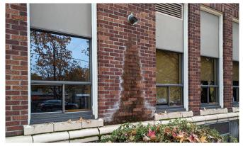
Figure 3.5.1 - Efflorescence at roof overflow outlet (cows tongue).
