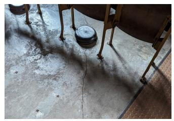
Figure 3.35.1 - Typical cracking, found throughout auditorium.
